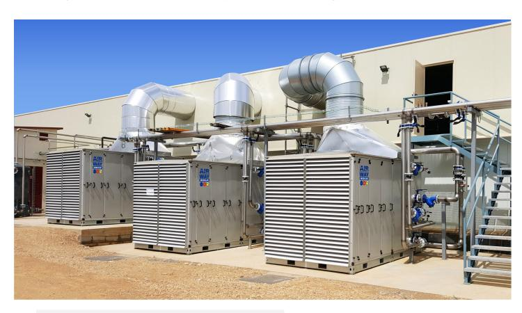
With its integrated PLC, the Modular system automatically manages the correct temperature, humidity, water flow and room pressures in the setter and hatcher rooms, creating the optimal environment for the incubation equipment.
